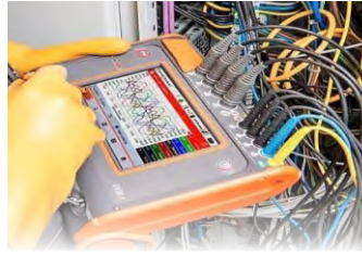
Greenfield Power Quality
