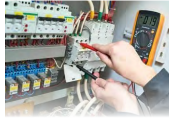
Electrical Safety Audit
